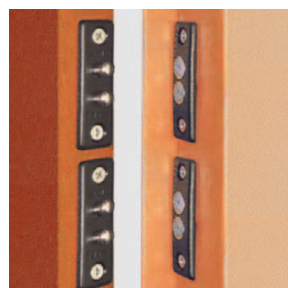
Double electrical contacts between leaf and doorframe
