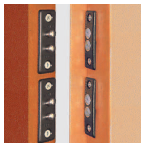
Double electrical contacts between leaf and doorframe
